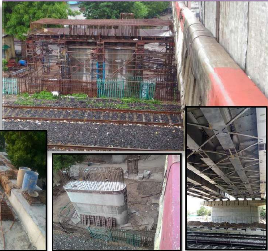
ACTUAL SITE PHOTOGRAPHS OF ROB EXTENSION
